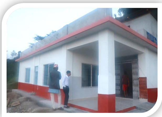
Finishing up newly constructed ward office
