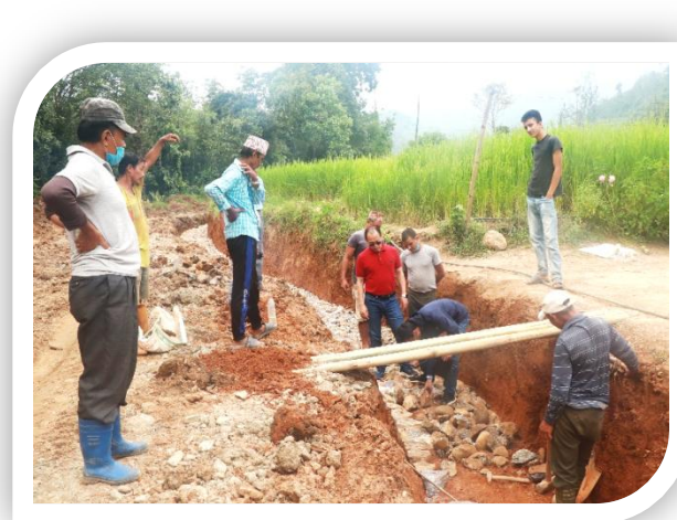
Inspection of road
